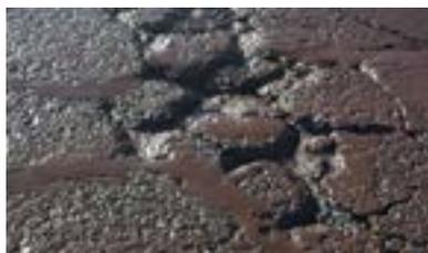
is why crack sealing is part of our annual maintenance. Potholes form when water works its way down into the road material and temperatures drop below freezing. The freezing water expands and causes a swell. When the tar that holds the road together freezes it becomes
